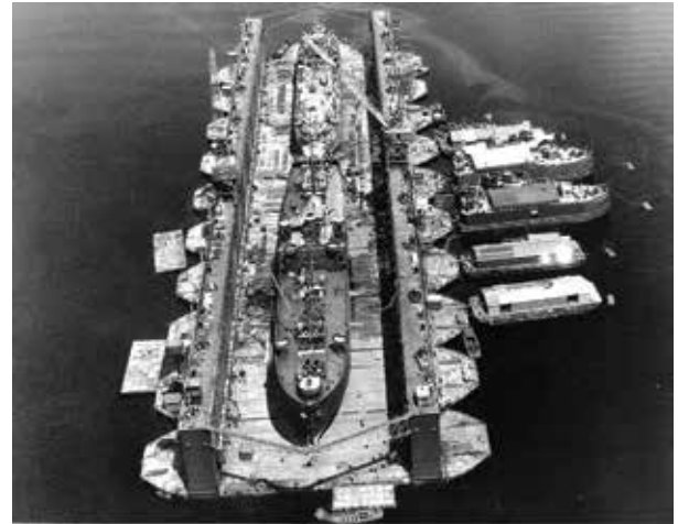
USS Artisan (ABSD-1) with Antelope (IX-109) and LST-120 in the dock at Espiritu Santo, New Hebrides Islands, January 8, 1945. The large auxiliary floating dry dock was built by Pollock in Stockton. U.S. Navy, Official U.S. Navy Photograph 80-G-314233, now in the collections of the National Archives.
